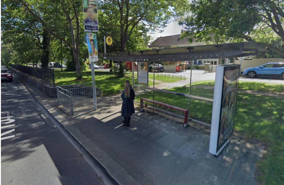
Figure 5: Footpath at Templeogue Road becomes too narrow for pedestrians to navigate for approximately 400m
