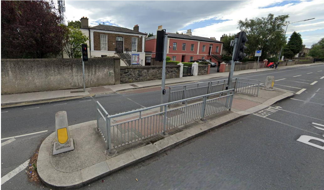
Figure 28: Pedestrian Crossing Point – Rathgar Road
