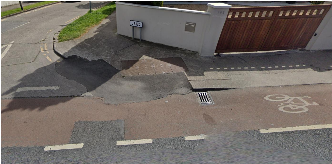
Figure 19: Surface Material - Rathfarnham Road
