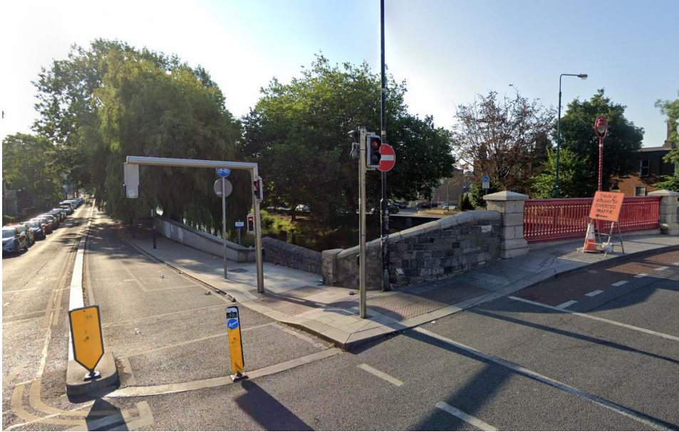
Figure 46: Shared Spaces – Richmond Bridge
