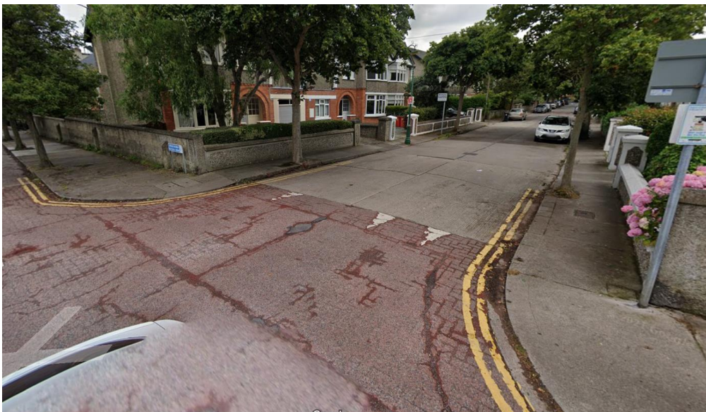
Figure 32: Uncontrolled Crossing on Victoria Road
