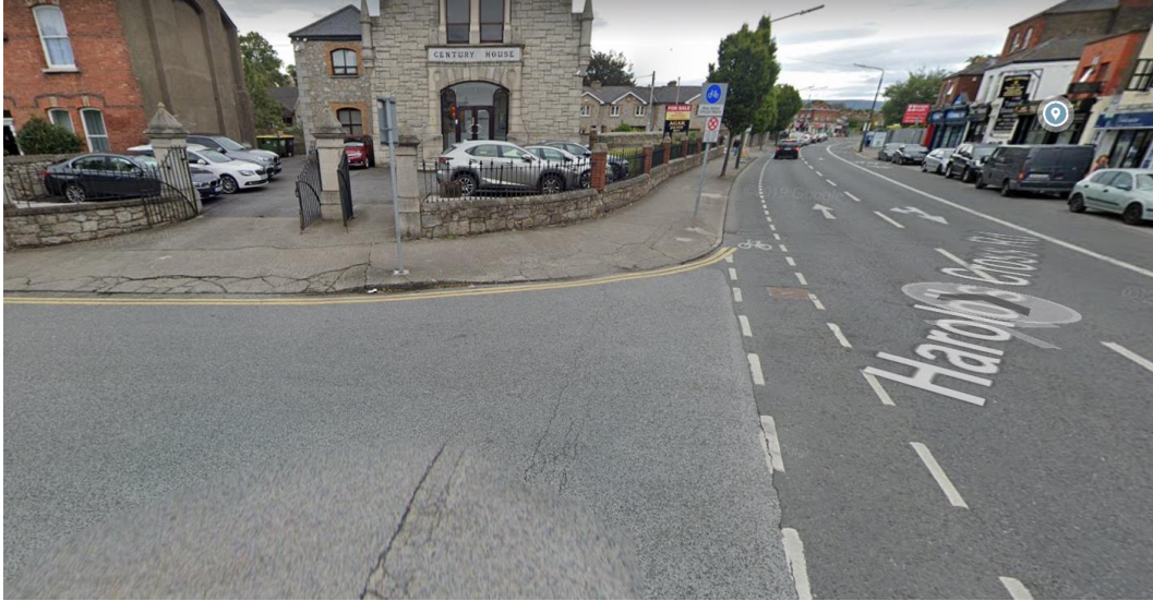
Figure 37: Surface Material on Harold's Cross Road
