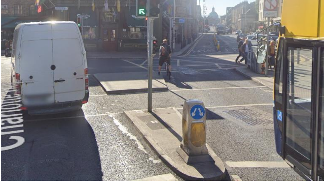
Figure 43: Controlled Crossing Point – Charlotte Way
