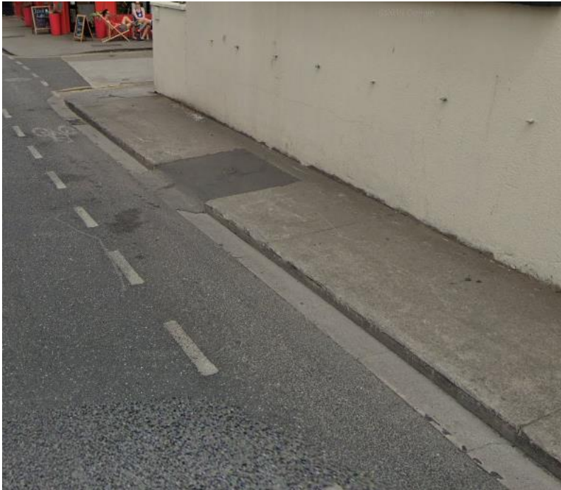
Figure 38: Surface Material on Terenure Road North
